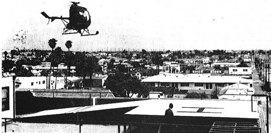
The minimum size (25' x 25') rooftop landing at California's Santa Monica Hospital is adequate for the smaller size helicopters.
